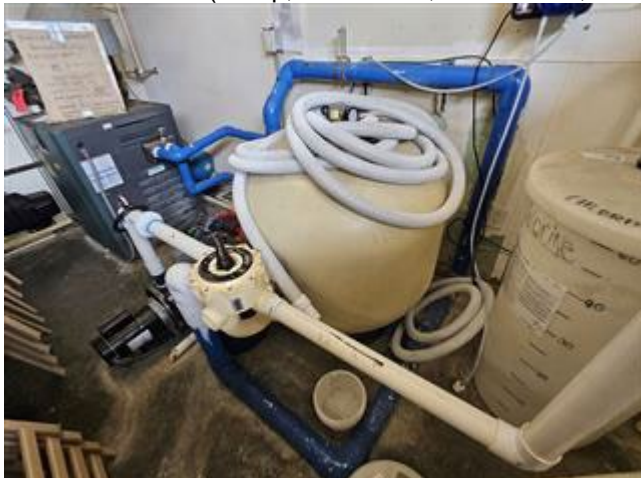
Pool Mechanical (Pump, Chlorination, Gas Heater, Filter, Pump Room Piping).
